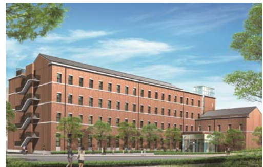
Hochikan Building (Graduate School of Brain Science) on the Kyotanabe Campus of Doshisha University
